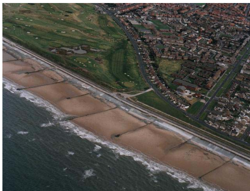
Rossall Point to Chatsworth Avenue
