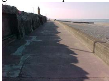
Five Bar Gate to Jubilee Gardens Unit 2/4/2
